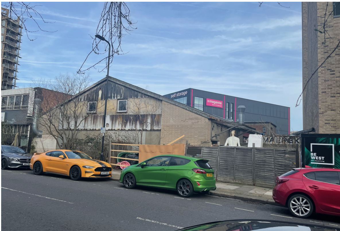
Figure 3: Application Site viewed from Bollo Lane
