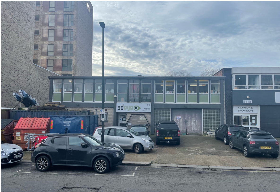
Figure 2: Application Site viewed from Stirling Road
